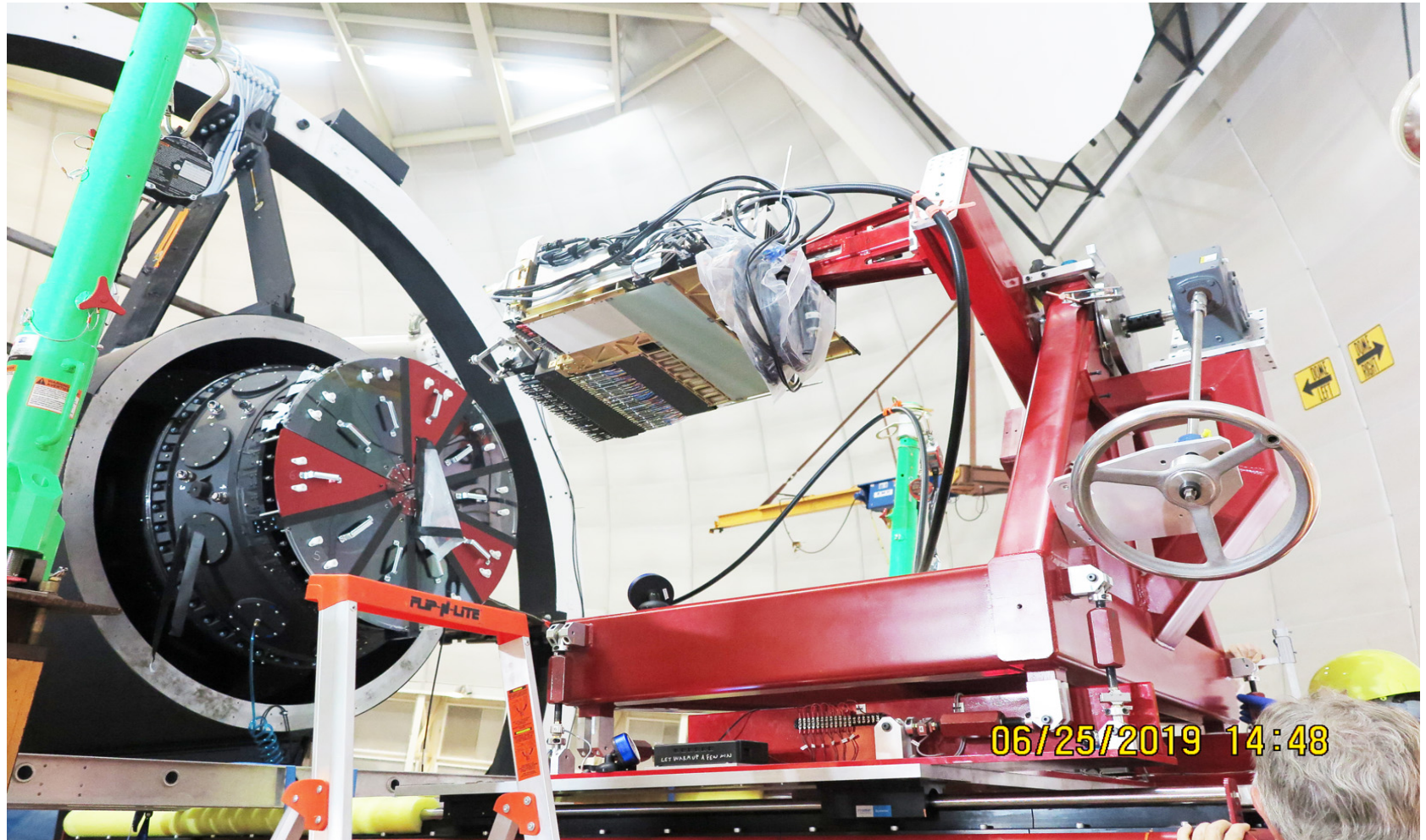
Petal is mounted to installation sled arm and slowly cranked into place
